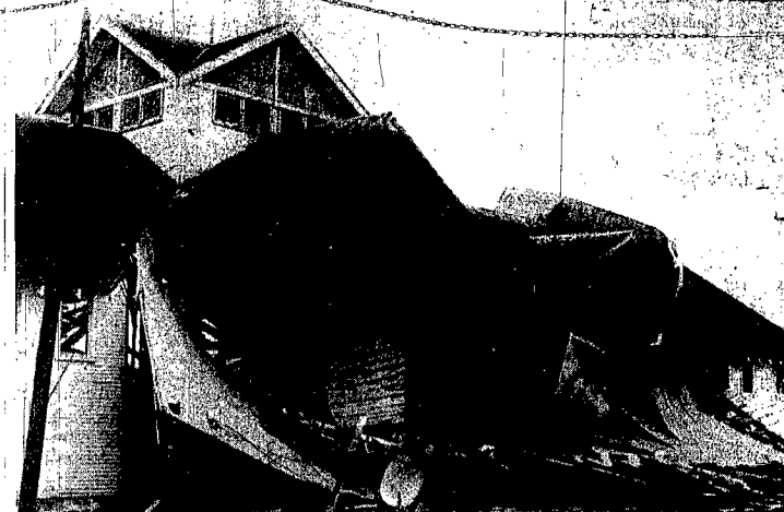
MONDAY'S HIGH WINDS took their toll at the Wayne County Fair grounds when the roof of the grandstand was blown off and smashed into the agricultural building. In addition to smashing the front of the building, part of the grandstand roof also cut into the ag building roof like a saw, as can be seen just back of the dormer windows near the end of the building.
